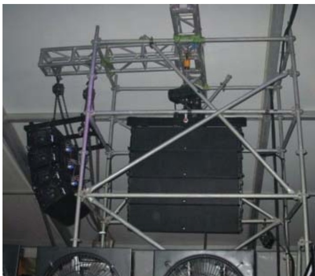
D.A.S. Audio flew in 8 units of Aero 38 line array systems (four for each side of the stage)
